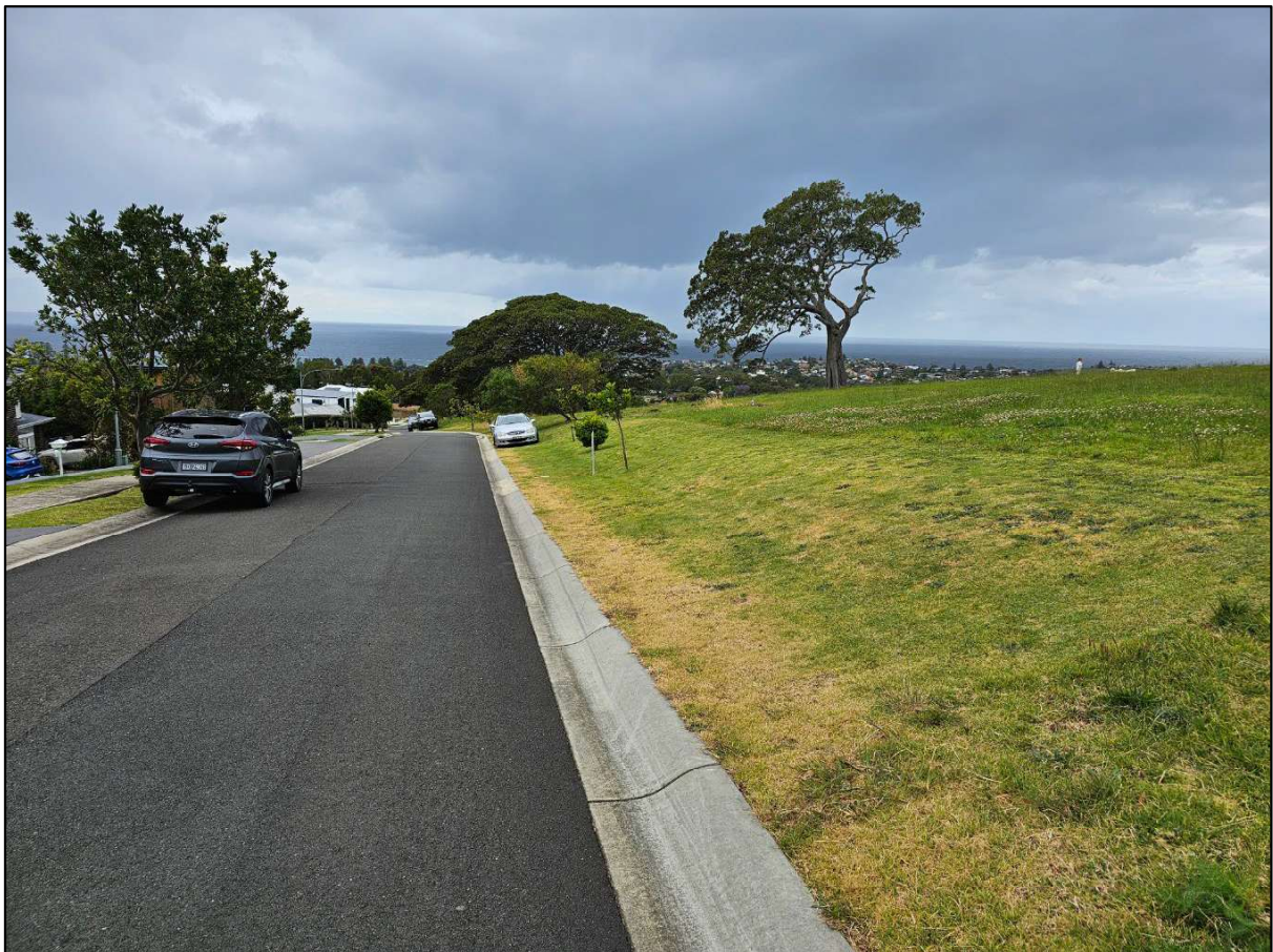
Photo 6 – View looking eastward down Caliope Street at the northern boundary of the subject site, noting the fully constructed road complete with kerb and gutter to the southern side.
