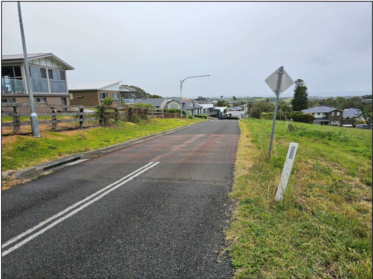
Photo 5 – Looking northward along Old Saddleback Road, at the western boundary of the subject site. Note the kerb and gutter along the western side of the road and unformed shoulder and verge on the eastern side.
